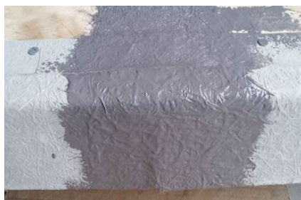
Double reinforced trim joint
