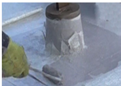
Local reinforcement to stanchion
